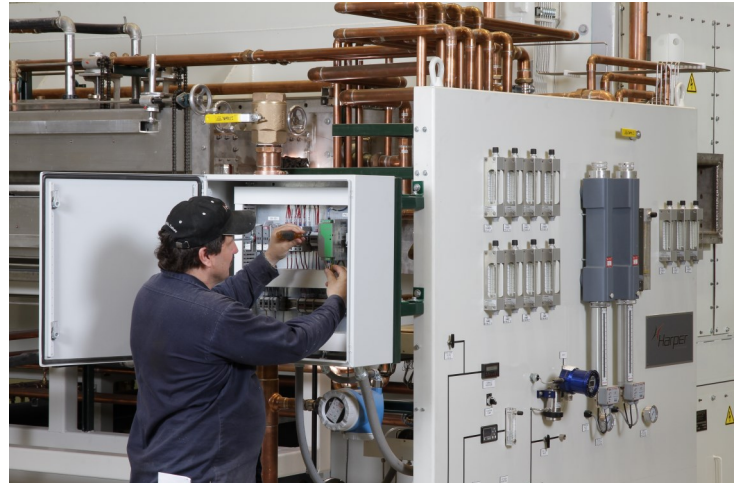
Image 1. The risk of partial or catastrophic failure can be greatly reduced by replacing and repairing at scheduled intervals based on time used or other measurable conditions.
